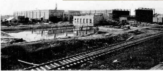
ARMY AND NAVY HELIUM GAS PLANT; ERECTED AT A COST OF $6,000,000
