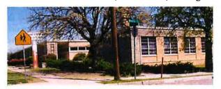
shape with the entrance situated at the southwest corner. The exterior is sheathed with yellow brick with irregular coursed rough-cut limestone used around the entrance and along portions of the south wing. Other design elements common to the era that are found on this building include the flat roof with overhang, wrought iron insets at the portico, and planters near the entrance. The
