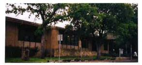
Epperly designed the U-shaped building. The 1-story brick building has a flat roof with a slight overhang above the windows. Aggregate panels are used below the window openings. Under the 1999 Bond Program, the school is scheduled to receive an addition of four classrooms, a computer lab, and other facilities. The contractor is ConReal Construction. Upon further assessment of its integrity, the school may be potentially eligible for the National Register in 2009.
